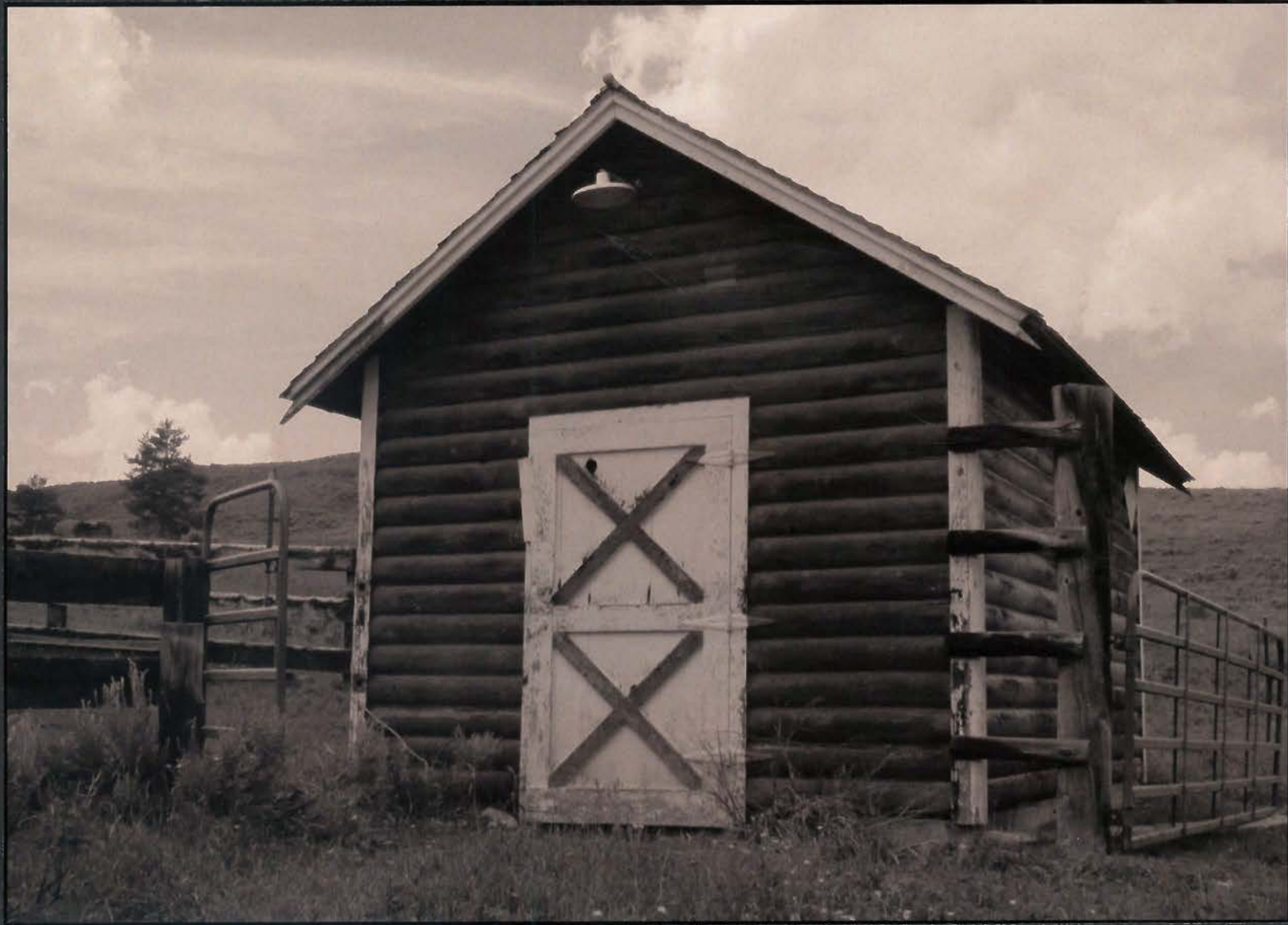
Looking northwest at the "Fly Shed" at Hoback Guard Station, 2017. Two such buildings were constructed here by the CCC in 1935, but the other was torn down.
