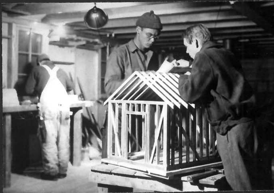
CCC carpentry crew trainees building scale model of camp building, Bridger National Forest, 1937. Photo courtesy MMM 2005.475.0001
