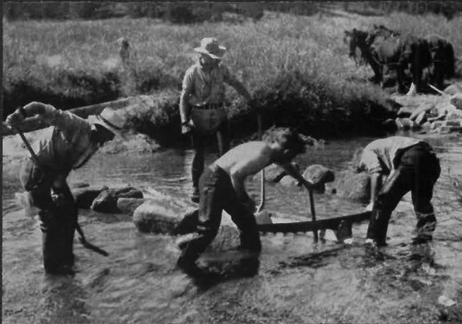
CCC crew building stream improvement. Montana, n.d. Photo courtesy forestarmyblogspot.com
