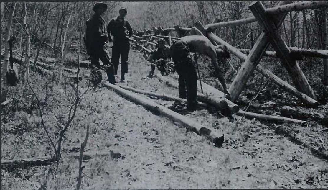
CCC boys building fence at Elkhart Park, Bridger National Forest, 1937.
