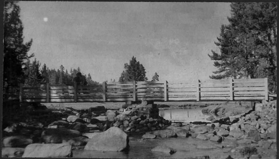
One of several livestock bridges built by the CCC over Big Sandy Creek, Bridger N.F., 1937. "Usually, at the season when stock is thrown on the Forest grazing lands, the waters of this creek are so high as to prevent movement of the bands." Photo courtesy MMM 2005.475.0001
