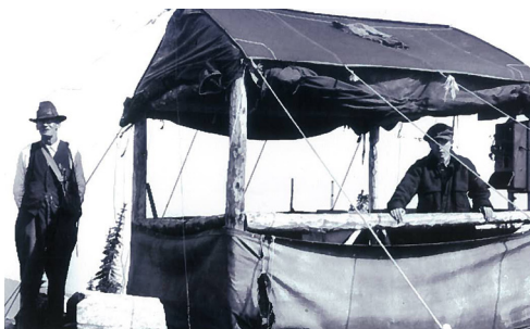
Elise Mountain lookout station (British Columbia, Canada) showing open canvas lookout shelter of frame construction and a telephone for communication. 1928. Photo used with permission from the Forest History Society, Durham, North Carolina, www.foresthistory.org .
